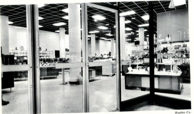
ISAAC HAM-BURGER & SONS DOWNTOWN STORE. Complete remodeling including designing all store fixtures. Area: 6,000 square feet. Mechanical Engineer: Henry Adams, Inc. Builder: Goodman Construction Company. The open aluminum t-bar ceiling was dropped below the existing ducts, sprinklers and electric conduit, which were all painted out black. Fluorescent panels and spotlights hung.
