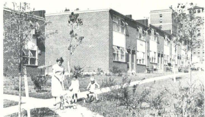
Johns Hopkins Garden Apartments Cochran, Stephenson & Wing
