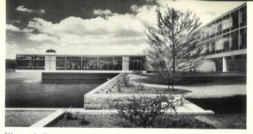
View of Connecticut General Life Insurance Company's new home office building looking west. Shown is the one-story cafeteria wing cantilevered over a reflecting pool and connected to the main three-story work level. The cafeteria has a seating capacity of 800.
