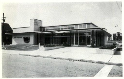
EUTAW SAVINGS BANK OF BALTIMORE BRANCH. Cost per square foot: \$29.11. Cost per cubic foot: \$2.36. Mechanical Engineer: James Posey & Associates. Structural Engineer: Alexander E. Forrest. Contractor: Cogswell Construction Company. Building prepared for future second story.
