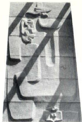
Precast sculptured 2½-ton wall panels. 2000 were used for Chicago's McCormick Place. Architect: Alfred Shaw, Chicago. Sculpture: Con- stantino Nicola.
