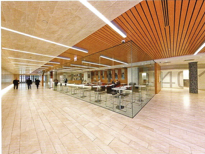
Griskelis Young Harrell redesigned the two lower levels of 401 N. Michigan, expanding amenity offerings and accommodating new building systems infrastructure.
