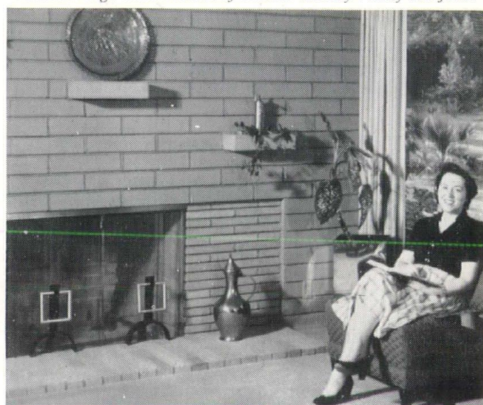
Raked horizontal joints add dramatic shadow lines to fireplace
