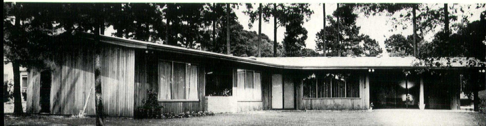
Exterior walls of heart redwood are used on rear elevation.
