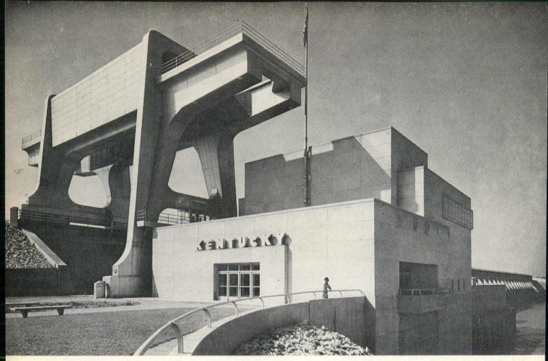
The greatest of all TVA dams—The Kentucky, completed in 1944 at a cost of \$119,200,000. It measures 8,422 feet, with a height of 206 feet, and approximately 7 million cubic yards of concrete, earth and rock went into its basic construction. The colossal gantry crane is the largest ever built by TVA and is one of the most attractive. Unlike any other TVA dam, Kentucky supports both highway and railroad.
