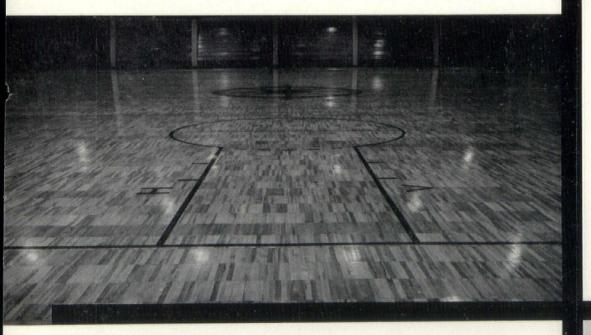
Ironbound is ideal. For extra protection against moisture absorption, swelling, shrinking, grain-raising, checking and *termites*, Ironbound is available treated with Woodlife by the Dri-Vac process.
