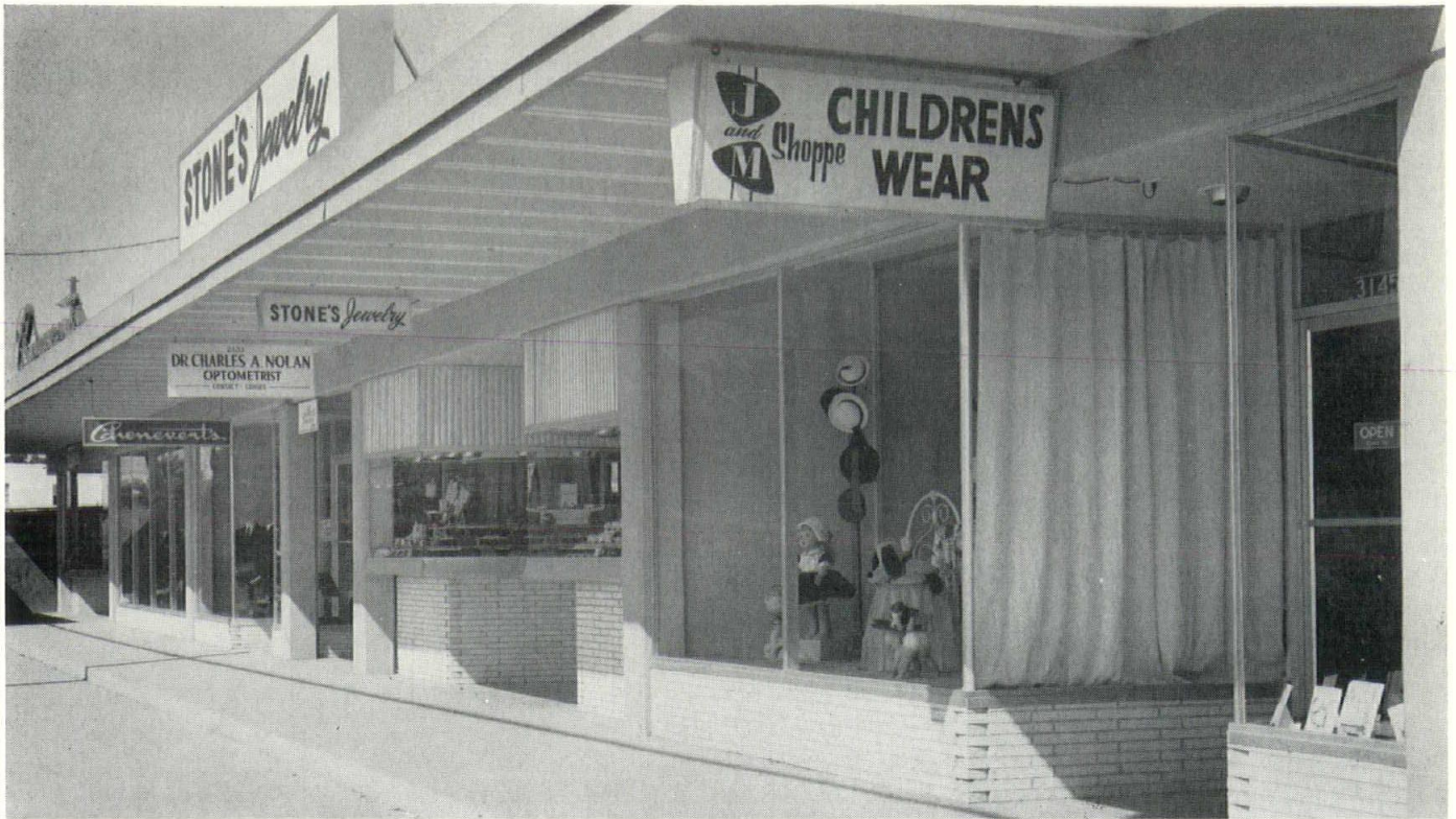
Photo of exterior of the Martinez Properties in Baton Rouge, Louisiana. A Hays Town Architect/Basso Plumbing and Heating Co., Mechanical Contractors.
