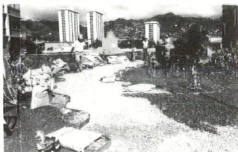
Area is prepared by forming a path to the width, length and thickness desired over suitable sub-base.
