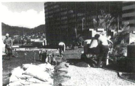
Epoxy-Rok is mixed — it is then added and mixed into the stones.
