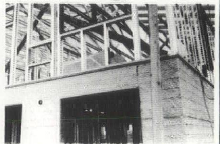
Paper-backed stucco-mesh on exterior metal studs.
