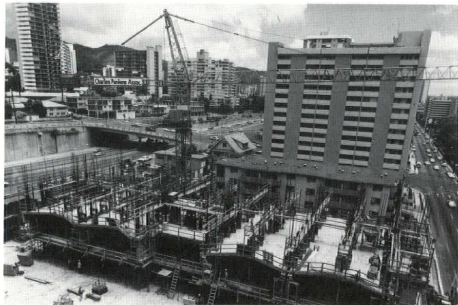
A slip form operation at Kinalau Tower.
