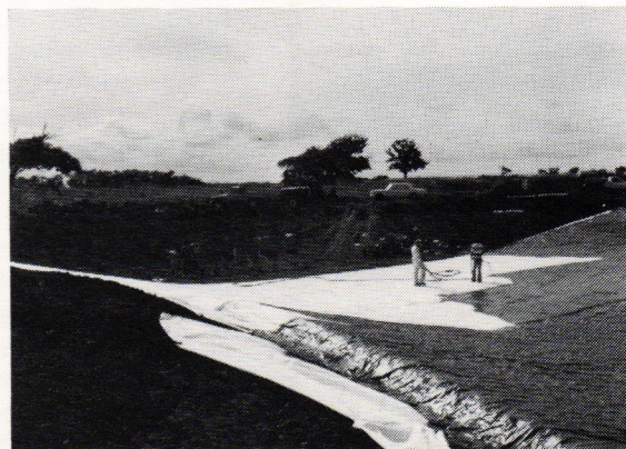
Polpu, Kauai - Chevron Industrial Membrane was used in the construction of this reservoir and water hazard for Kiahuna Golf Course. The spraying covers another product called Supac® which lines the area.
