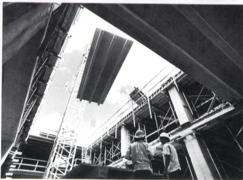
Erection of Tri-Tees at Kotake industrial/office complex on Waiakamilo Road, Honolulu. Walker-Moody Construction Co., Ltd., builder; Gerald Tokuno, AIA, architect; Martin, Early, & Bravo, structural engineers.
