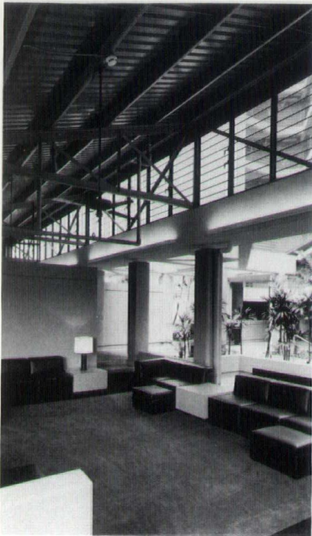
Natural ventilation was a primary consideration in building design. Many of the interior walls in the lounge area do not extend to the roof. Photo by Augie Salbosa.
