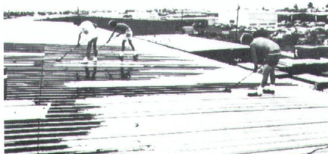
Kahului Maui — Chevron Industrial Membrane was used to seal the metal roof for the Haleakala Transportation & Warehousing facility.
