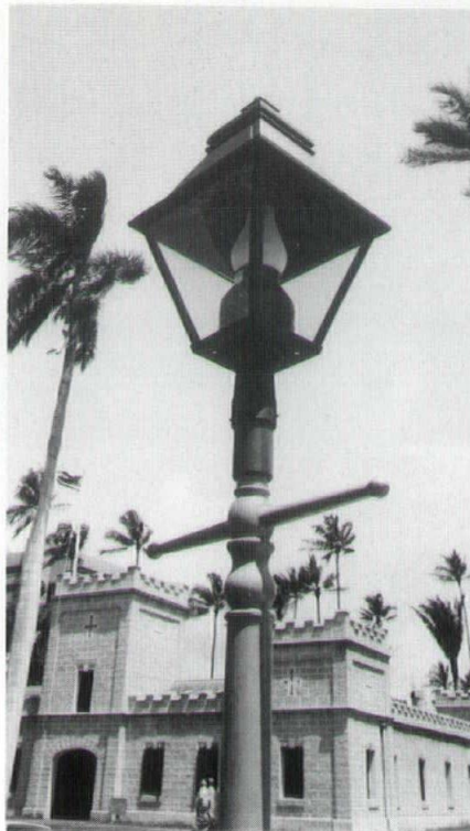
Cast iron lamp posts and reproduction light fixtures have been installed. They are replicas of posts and fixtures seen in period photographs.
