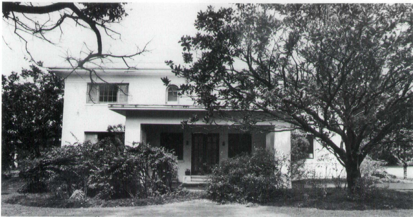
The two-story Sumner residence was designed by builder C. W. Winstedt in the early 20th century. The classically styled home is constructed of stuccoed concrete exterior walls and wood framed interior walls and floors. The flat roof, heavy cornice and massive walls give the home a forceful presence which is accentuated by the heavy porte-cochere over the main entry. The house is basically "U" shaped in plan with the first floor rooms wrapping around a large semi-enclosed lanai, allowing almost every room to have generous exterior exposure. Photo by Phil Spalding III.
