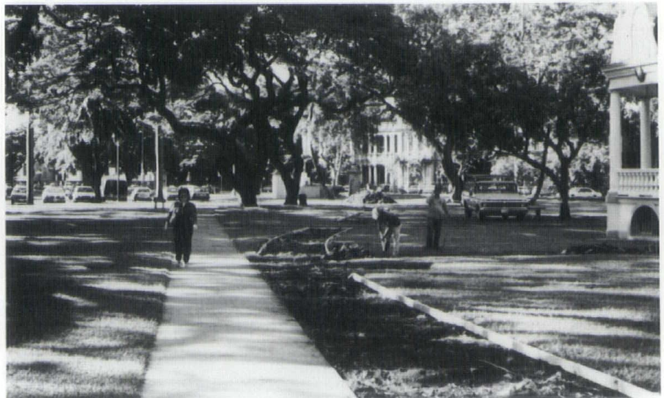
New concrete walkways are colored and textured to resemble the rolled black sand used originally. Construction was scheduled to minimize impact on public access to the palace.
