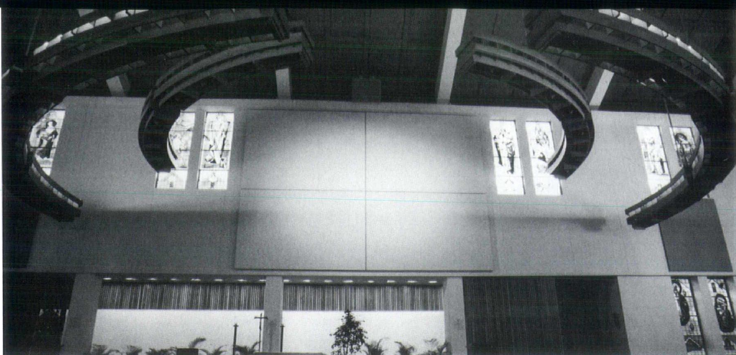
Concentric wood rings with neon lights are segmented into 12-foot arcs with monopoint floodlights underneath in each bay.
