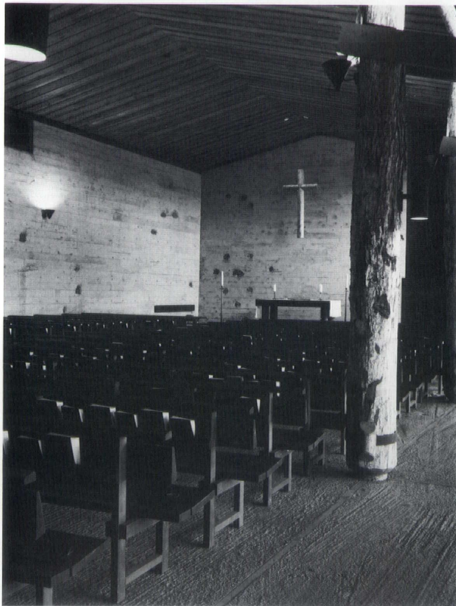
Ohia tree trunks are used as supporting columns in the chapel at Hawaii Preparatory Academy.
