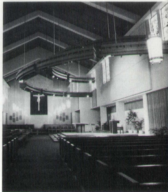
Gothic lanterns provide general lighting at the Co-Cathedral of St. Theresa. Two concentric wood rings provide accent lighting.
