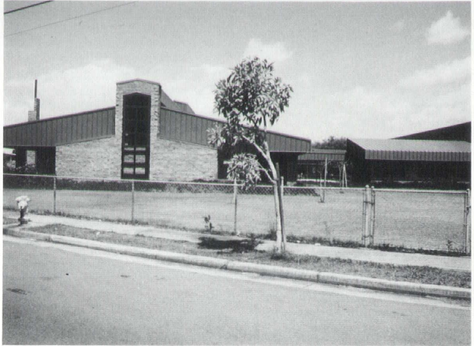
The Ewa Beach Chapel by CJS Group, Ltd. uses a continuous roof ventilation monitor to enhance natural ventilation and create a major form element.
