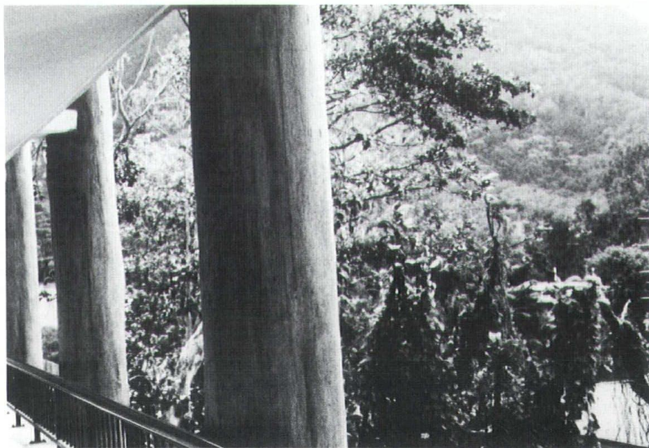
The Ramada Reef Resort, nestled in a grove of ancient palms and melaleuca trees, was designed to be a part of the forest. Columns of stained concrete were cast in a mold made from a rose gum log, giving them a tree-like appearance. Photos by Kevin N. P. Chun.
