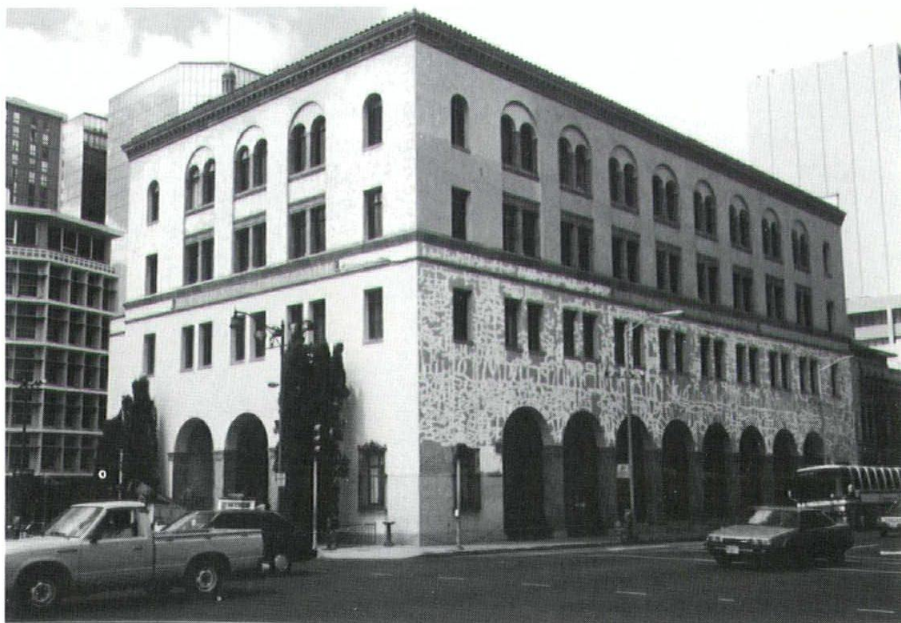
The Hawaiian Electric Company (HECO) Building, completed in 1927, was erected entirely without the use of wood. (Above) Reinforced concrete, hollow-tile and ornamented metals were used as the basis for construction. Sixty years later, HECO received a functional weatherproofing facelift. (Below) Comparing both photos, note how cracks in stucco conform to joints in hollow-tile blocks. Photos courtesy of HECO Corporate Library
