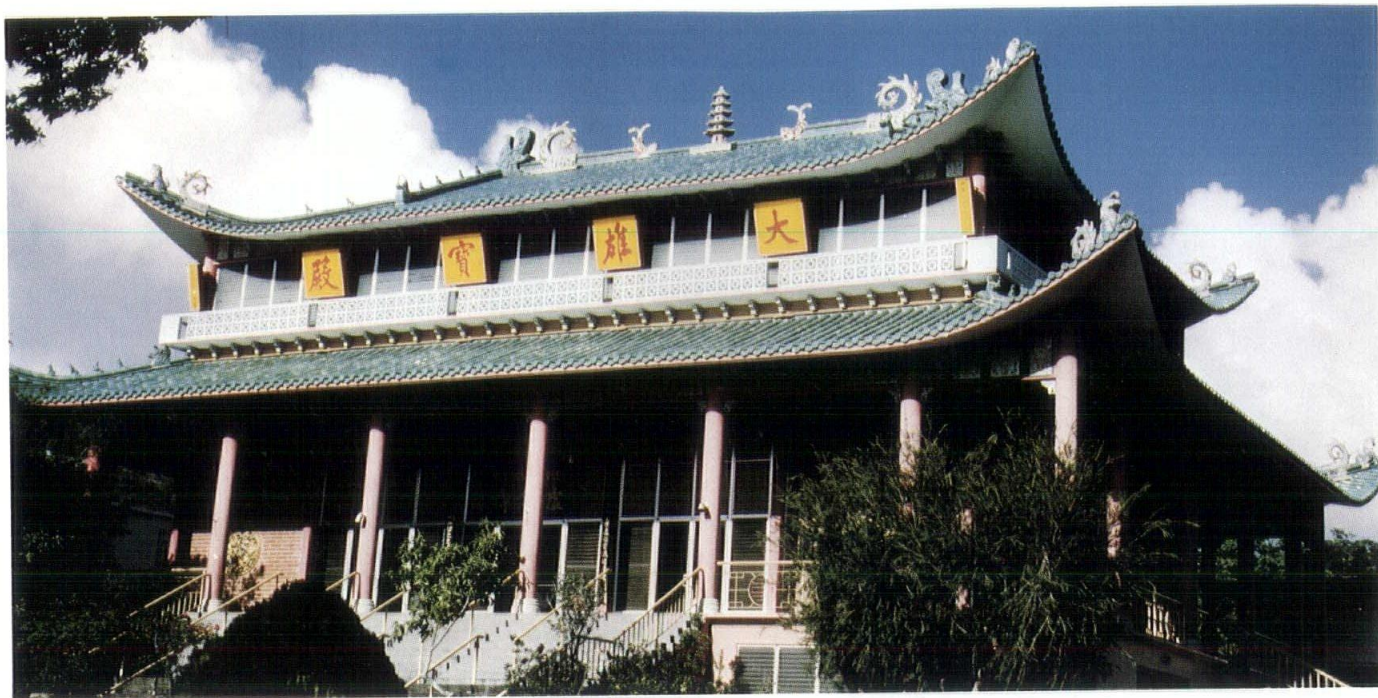
A two-piece Chinese clay roof was brought in from the Orient for this picturesque house of worship, the Chinese Buddhist Hsu-Yun Temple. Installed by Honolulu Roofing, all of the tile and ornaments in this unique configuration were attached with cement. Photo by Philip Spalding III
