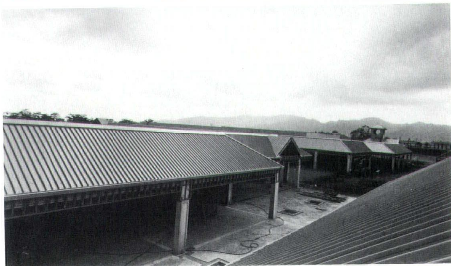
(Top photo) A close up look at a "clip down" metal roofing system being used at the Mililani Town Center (above) now under construction in Central Oahu.
