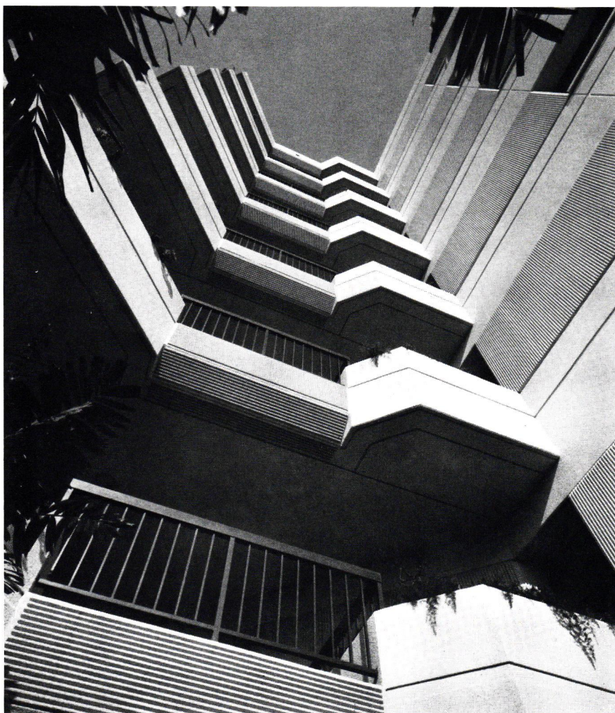
An exterior view of the Queen Emma Tower shows the combination of precast and poured-in-place ribbed formed concrete contrasted against smooth, poured-in-place horizontal bands of concrete. Photo by Augie Salbosa
