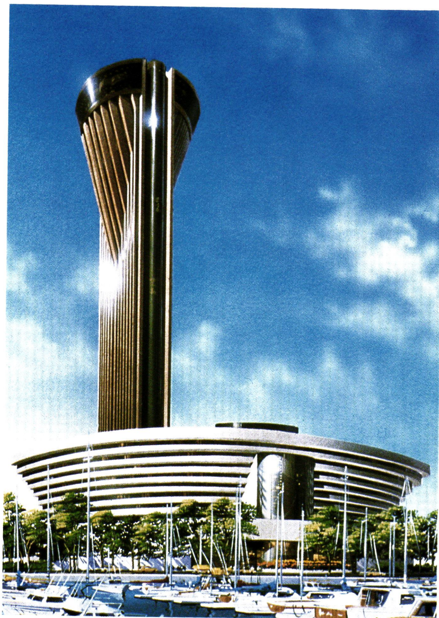
At Marina Center Complex, Singapore, curved concrete cantilevers and large shear walls were used to achieve the final design.
