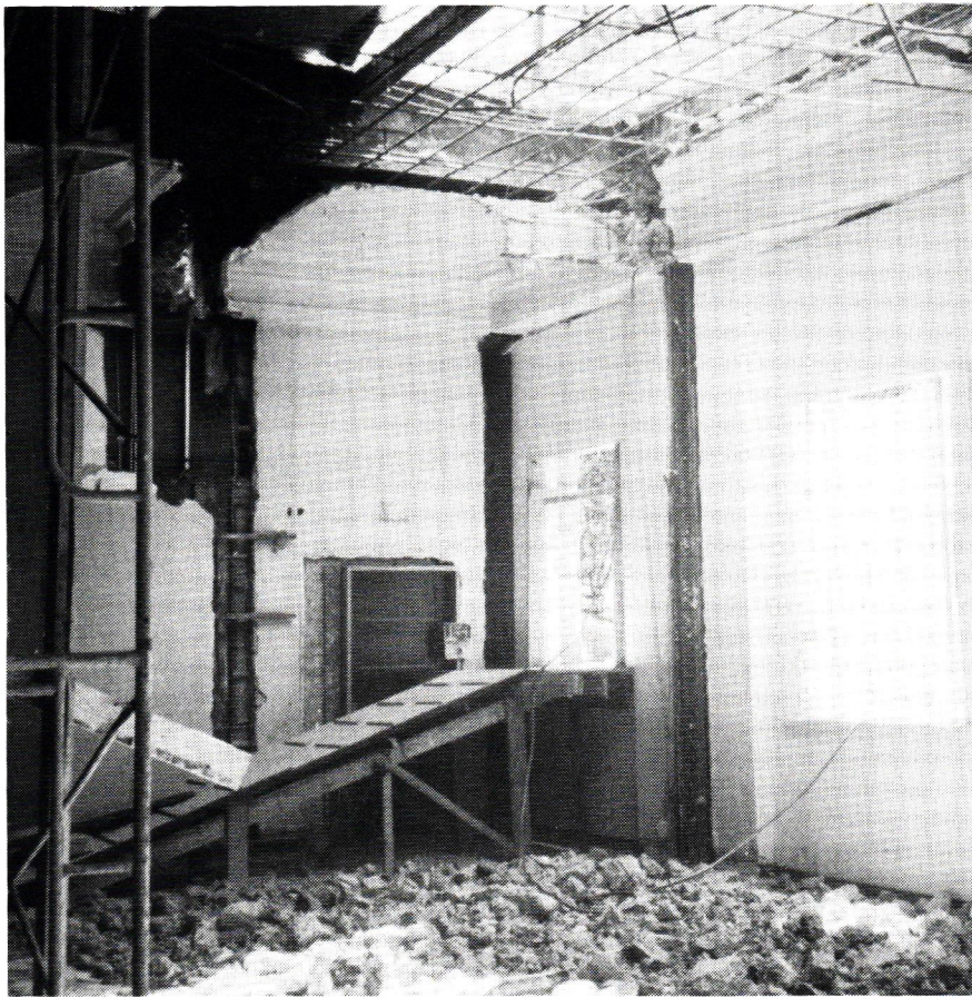
The Supreme Court takes on the appearance of downtown Beirut as layers are peeled off to expose what is left of the early 20th century walls and ceiling. The court room will be renovated in early 20th century character using original elements which are able to be salvaged.
