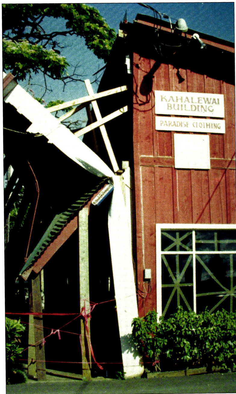
The facade completely separated from the roof assembly of the Kahalewai Building leaving it to lean perilously over the sidewalk for months before repairs were completed.
