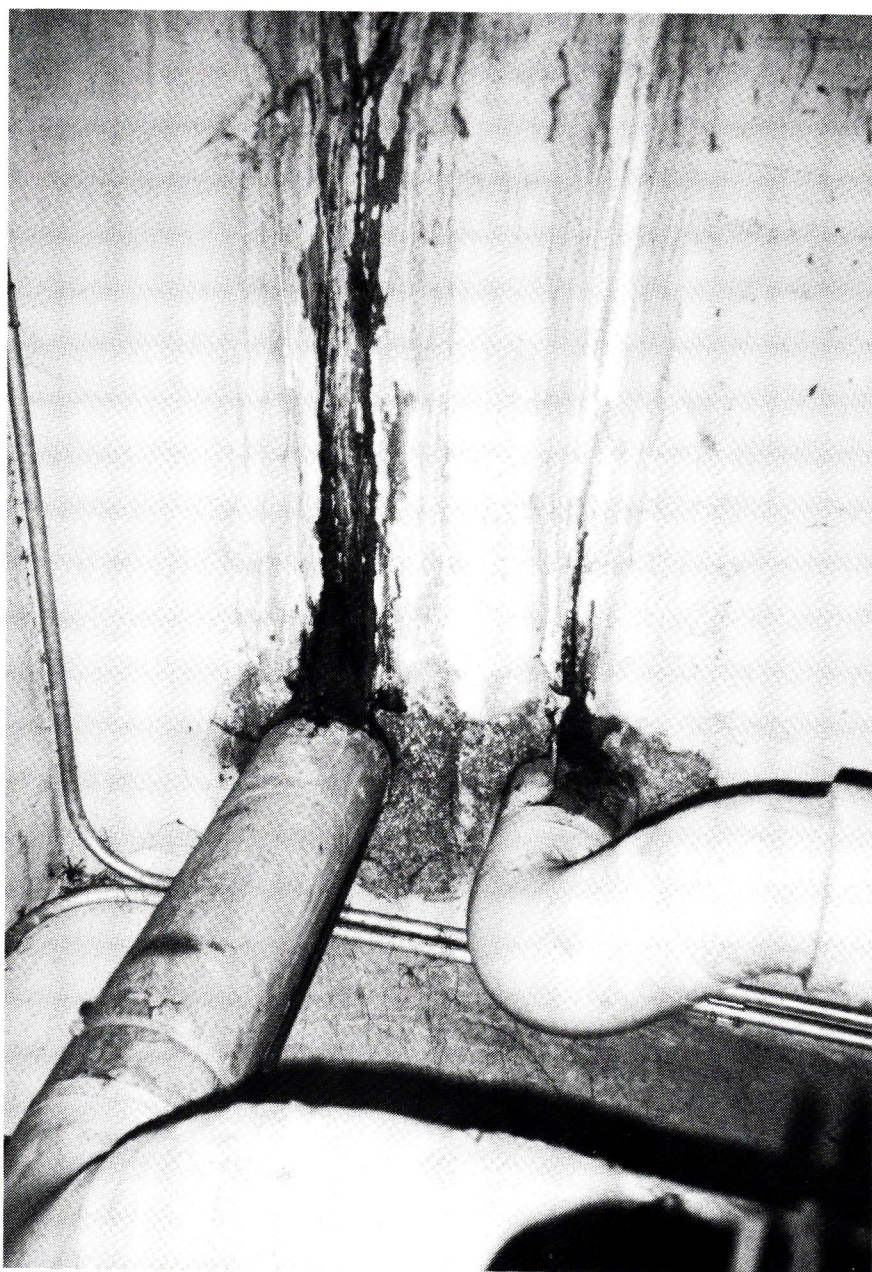
Wall penetrations not properly waterproofed can result in constant water leakage into a structure and outside spalling.
