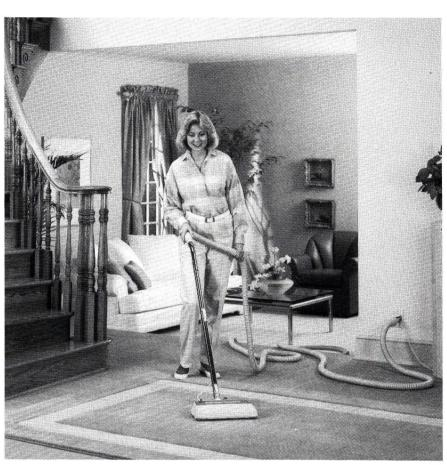
A flexible hose connected to a wall inlet pulls dirt into a central vacuum cannister installed away from living areas in a home.
