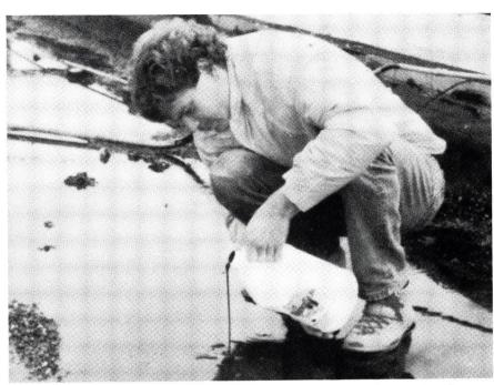
Seek & Seal can be poured full strength into standing water to repair cracks up to ¼ inch wide.
