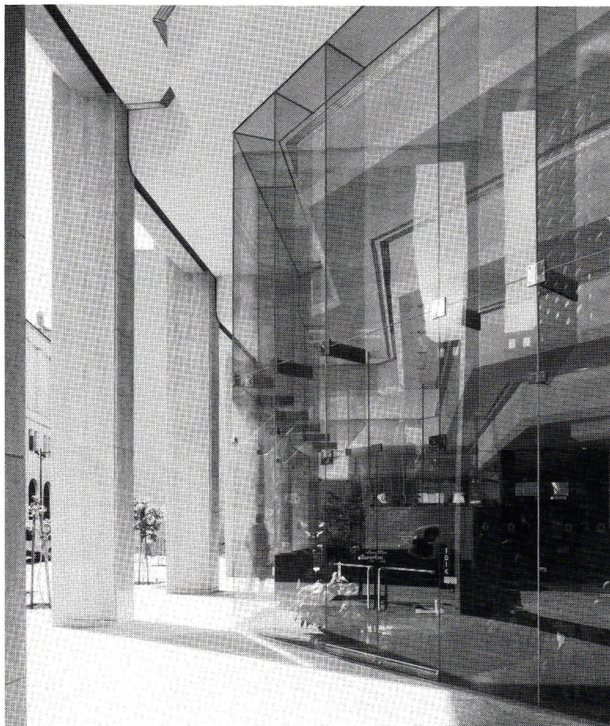
The design concept of City Financial Tower, one of the last architectural efforts of the late Minoru Yamasaki, is to eliminate vertical framing elements. Glass is sealed with glass caulking and steel gaskets.
