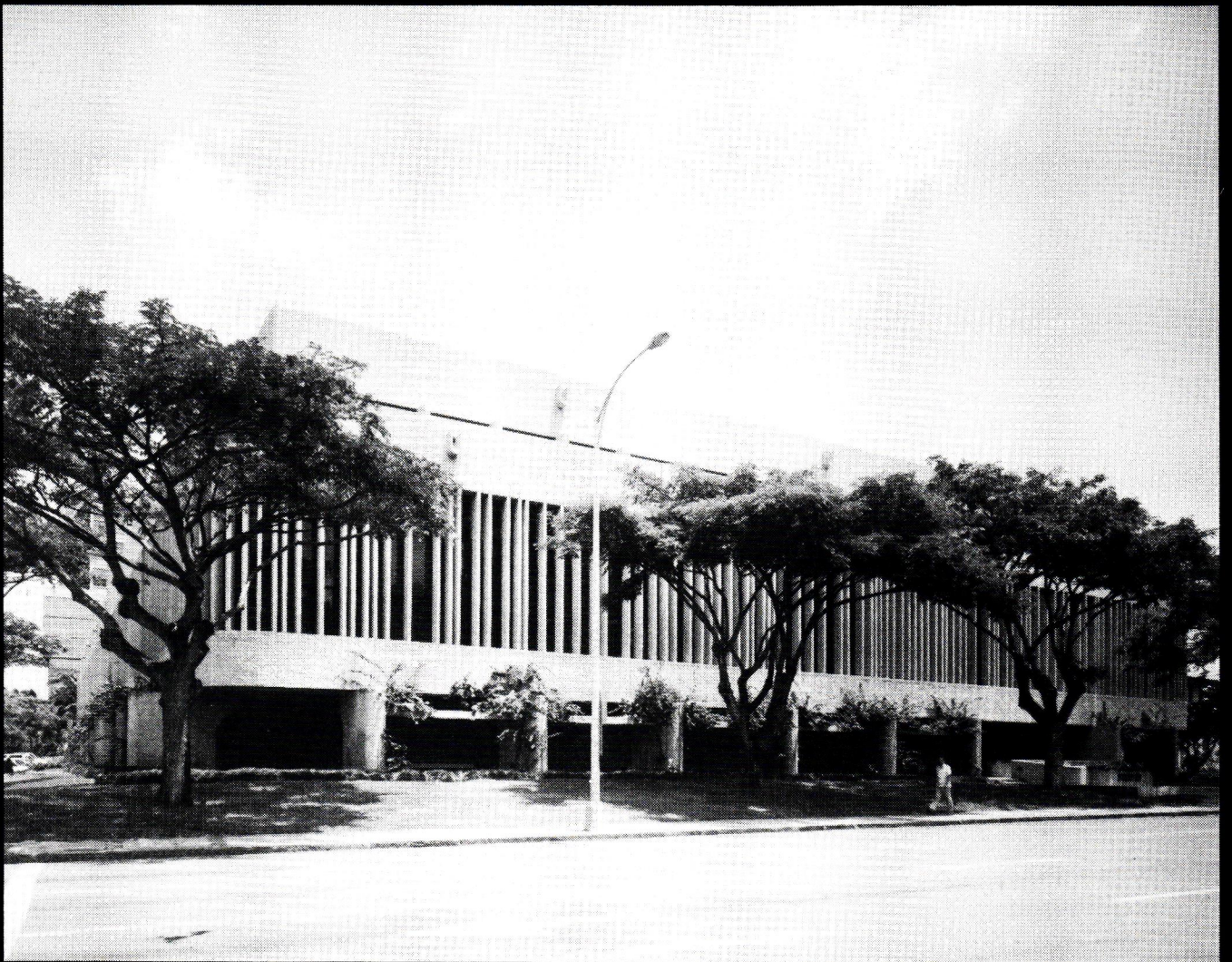
This view of Keelikolani Hale from the corner of Punchbowl and Halekauwila streets shows the four-story office structure with precast concrete panels and vertical pins. Photo by David Franzen
