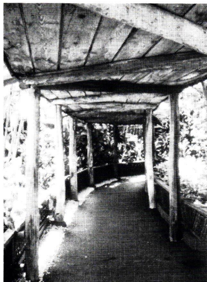
In the entry breezeway path and roof, viewed here from the Hausten Street entrance, beams of ohia follow a zig-zag pattern in framing the roof. In plan the path is an arc. Posts and beams connect via a peg of smaller diameter wood. Photo by Sid Snyder
