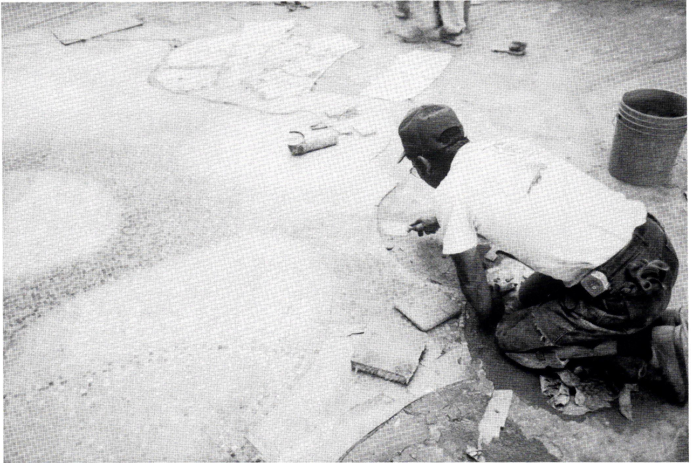
Use of paper-backed sheets and the jigsaw puzzle nature of the installation were among the unusual characteristics of renovating the mural.
