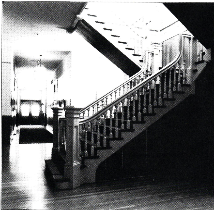
Above and below: Before and after shots show historically accurate restoration of the grand stairway. Original handrails and balusters were salvaged and used to rebuild the stairway.
