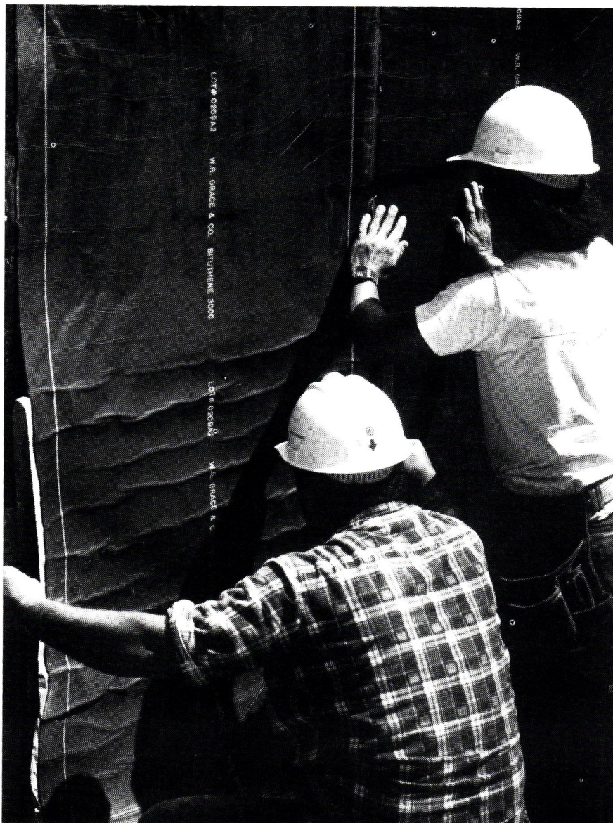
Field technicians at Grace Pacific Roofing install sheet waterproofing and protection board on a below-grade vertical foundation wall at the construction site of the Queen's Medical Center office building. Photo by Camera Hawaii
