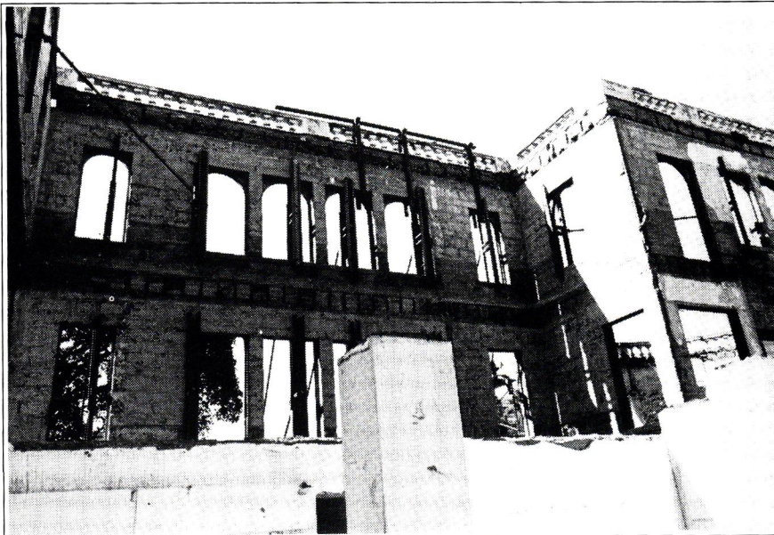
Above: For some time after demolition, all that remained standing of the original structure were the exterior walls. Below: Original walls were not reinforced, and extensive stabilization measures were necessary in the reconstruction.
