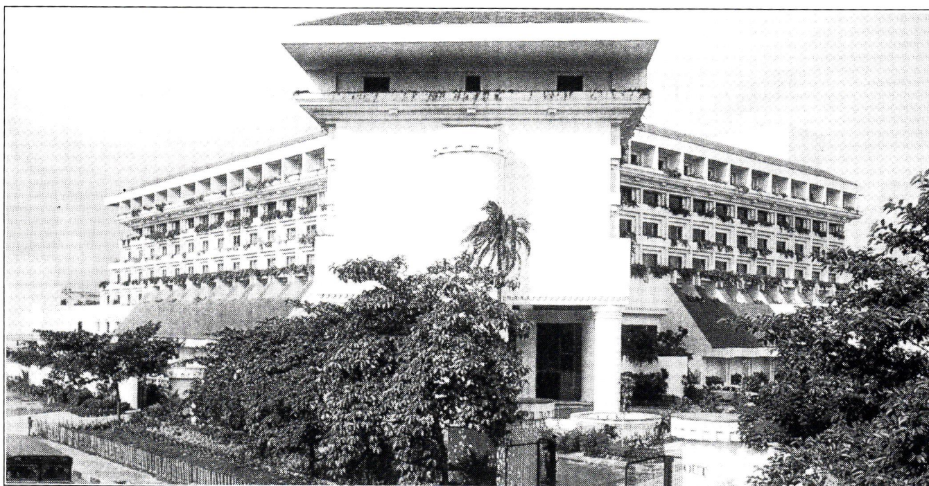
Above: Design of the hotel incorporates many elements found in the Calcutta area, including relief details, planters and stepped window frames. Below: The Taj Bengal's triangular design allows security guards a clear line of sight to all doors at each level.
