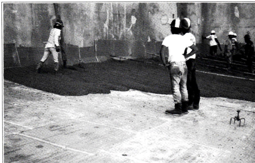
Volclay Bentonite panels are installed on grade before rebars and concrete.
