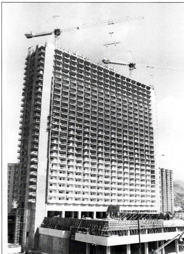
Novel construction techniques utilizing Yee-developed splice sleeves were used for the first time in the 38-story Ala Moana Hotel.
