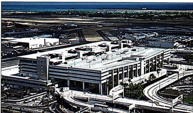
Thermo-plastic single-ply roofing was chosen for the Interisland Terminal at the Honolulu Airport due to its superior seam strength and resistance to UV rays.
