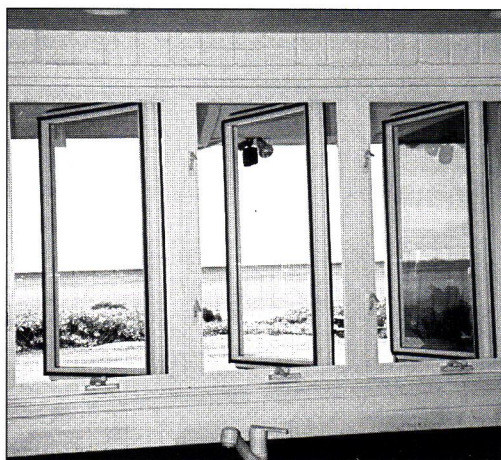
Casement windows can catch the air moving parallel to the outside wall and direct its movement inside a structure.
