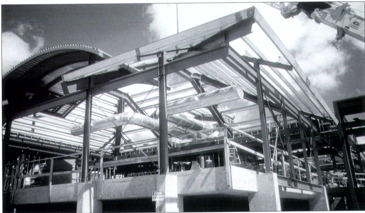
The hip roofs are made of prefinished metal roof panels on gage metal purlins.
