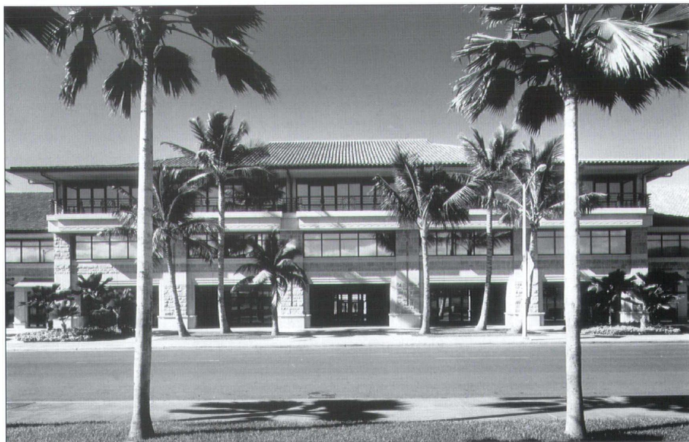
Split-faced granite and honed limestone were chosen to convey an image of quality with the Campbell Building.
