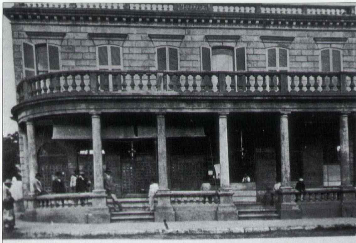
Opened in 1871, the Kamehameha V Post Office was the first all-concrete building in Hawaii.
