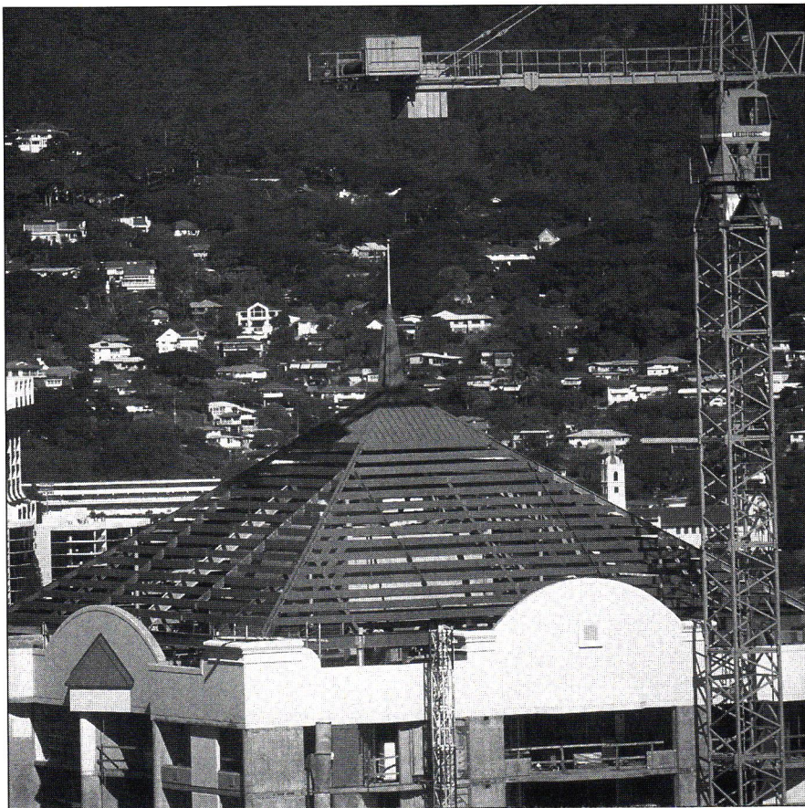
A steel roof trellis completed the 41-story tower at One Archer Lane.
