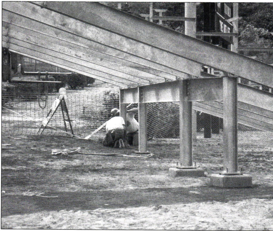
Concrete footings provide the foundation for the steel structure.
