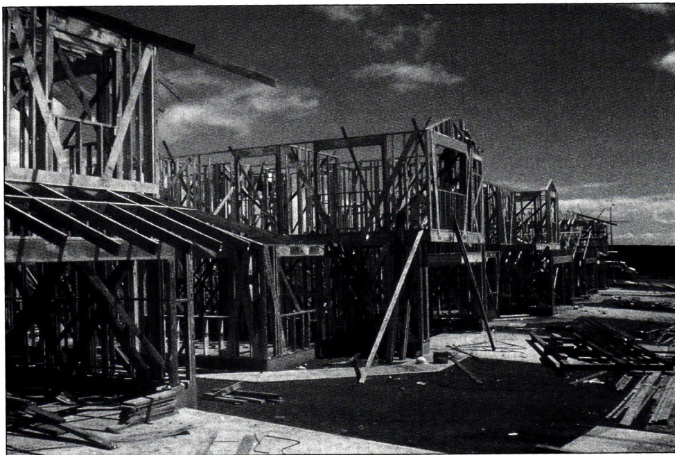
Developer Castle & Cooke's new subdivision at Mililani Mauka features thousands of homes framed with steel.
