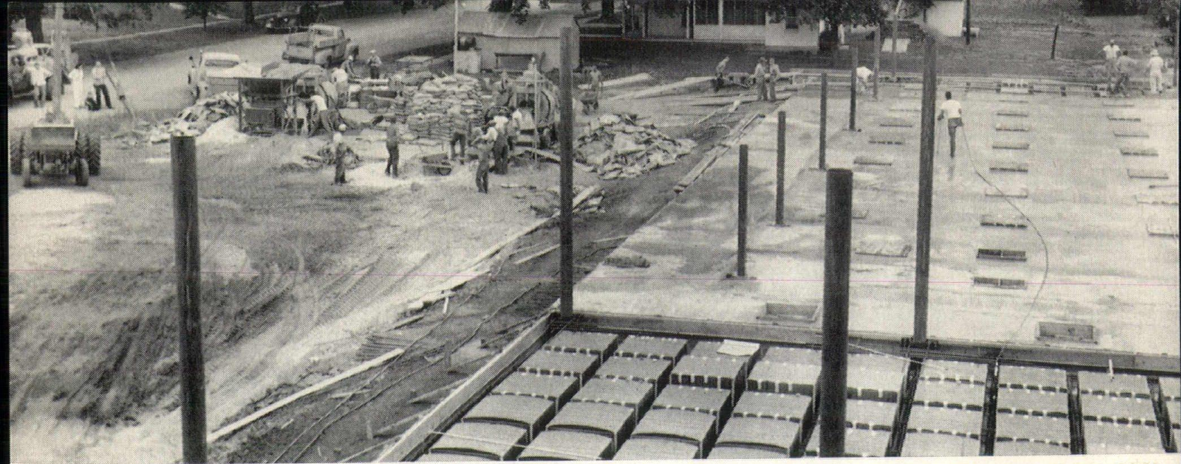
SECOND DAY OF CONTINUOUS POURING FINISHES CLASSROOM SLAB, REAR. FOREGROUND, BOX MOLDS WILL FORM GRID IN GYM ROOF.
