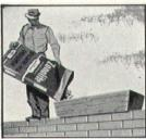
Filling blocks or cavities is easy. Sometimes, a simple hopper is used to facilitate installation.
