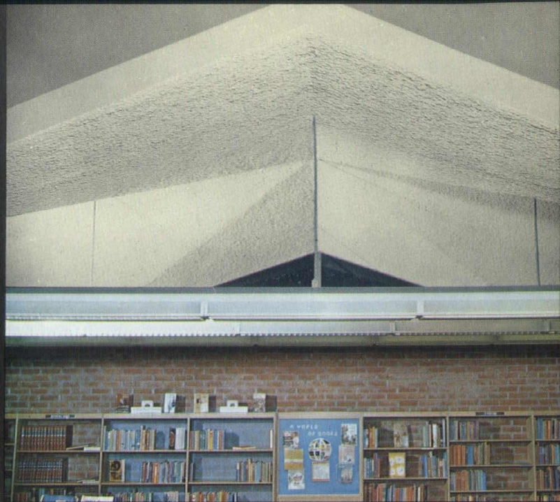
SOUND ABSORBING texture of Hi-Sorb is clearly defined in this acoustic ceiling in the Los Angeles Library. Architects: Bowerman & Hobson.
