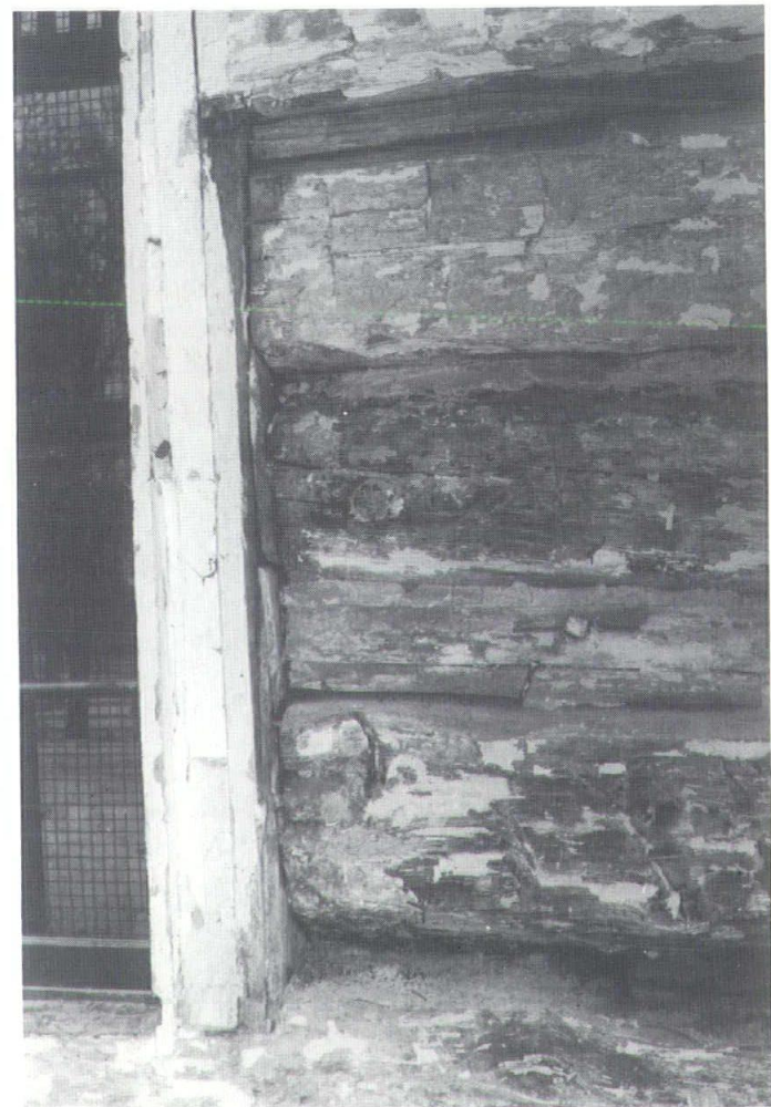
C. Original window jamb notched into beams was left in place when new opening was made.
