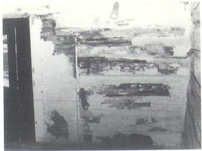
B. South wall of cabin showing original main door opening uncovered during investigation.
