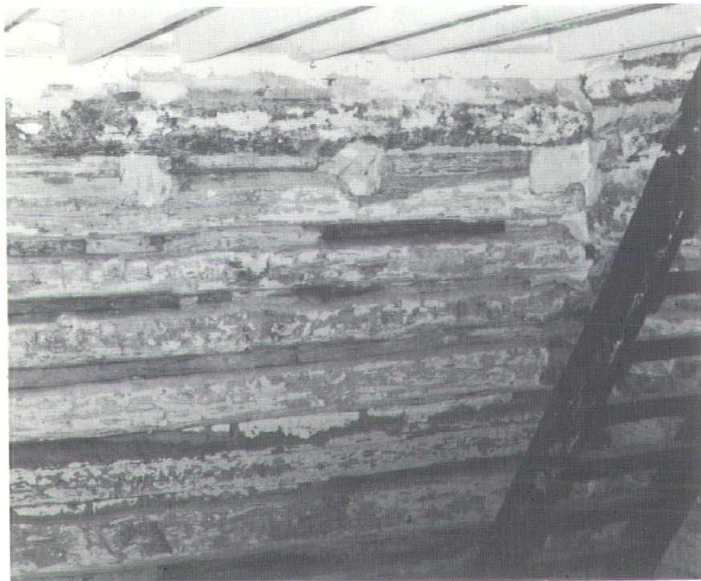
A. North wall of cabin showing location of original loft floor beams.
