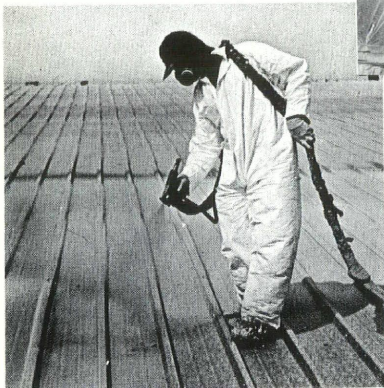
Application of Isofoam urethane to roof
