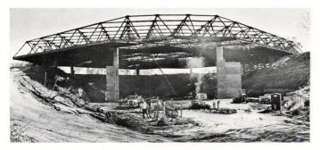
A 420 x 378-ft rectangle with clipped corners, the 26.5-ft-deep truss in plan resembles the seams of a patchwork quilt. The main repeated unit is 42-ft square weighing 18.4 psf, formed by four wide-flange bottom chords, 27 in. deep. Round tubes 12 in. In diameter, some with fins, are used for both the diagonal web members and the skewed upper chords. If the upper chords were in the same plane as the wide-flange beams, they would inscribe 29.5-ft-sq diamonds in the bottom squares.
