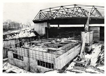
The arena is being nestled into a natural, 50-ft-deep ravine that only had to be excavated by about 10 ft and widened. A clear glass curtain wall will cover the 15-ft-tall above-grade portion of the arena, which spills out over the edge of the bowl and includes entry and access areas. The structure's, long-span steel roof is now in place. It is the patented Takenaka truss—a space truss with its top chords skewed 45 deg from its bottom.
