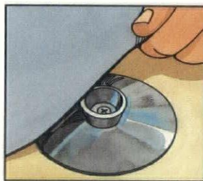
1 Roll membrane over knobbed base plate.
