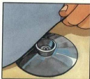
1 Roll membrane over knobbed base plate.
