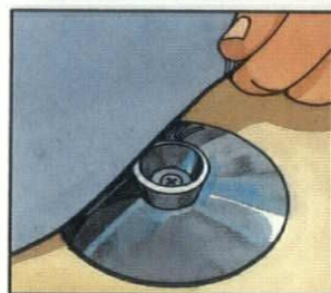
1 Roll membrane over knobbed base plate.
